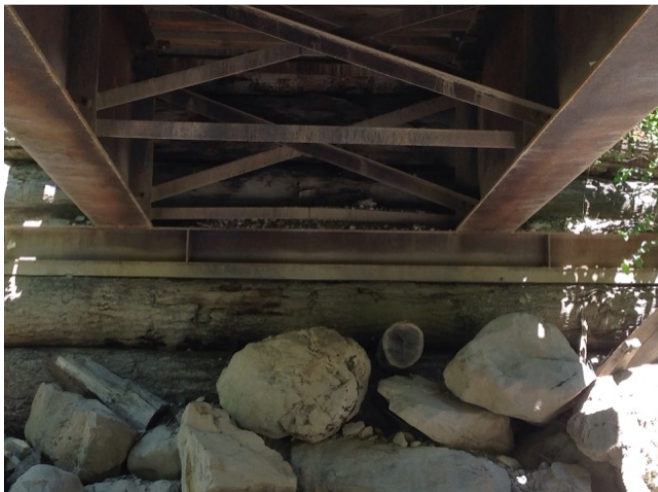
Right Bank Abutment when facing downstream
