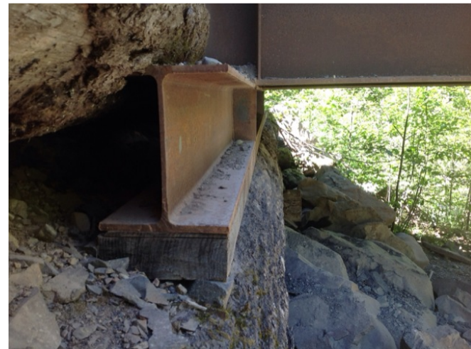
left bank upstream bearing
