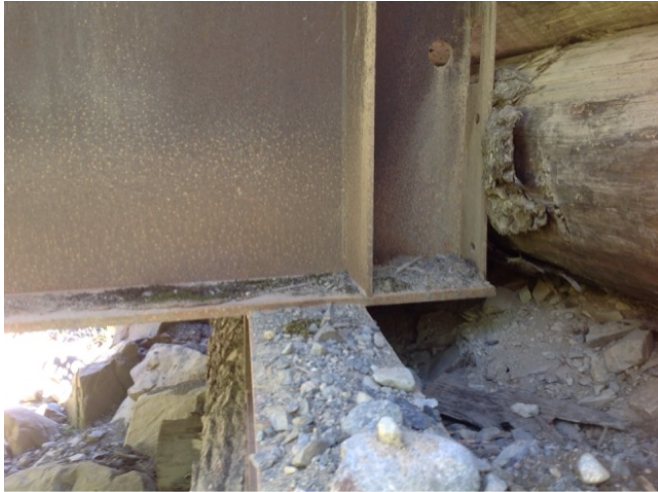
left bank downstream bearing
