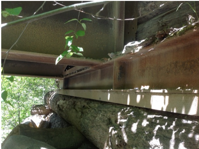
right bank bearing
