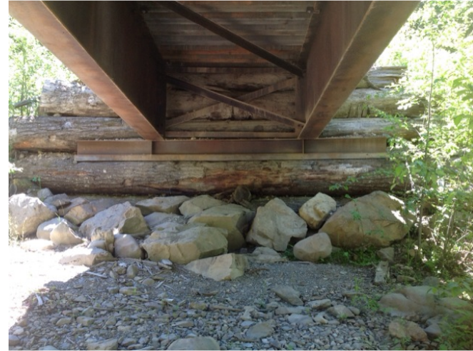
Left Bank Abutment when facing downstream
