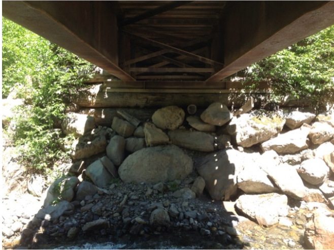
Right Bank Abutment when facing downstream
